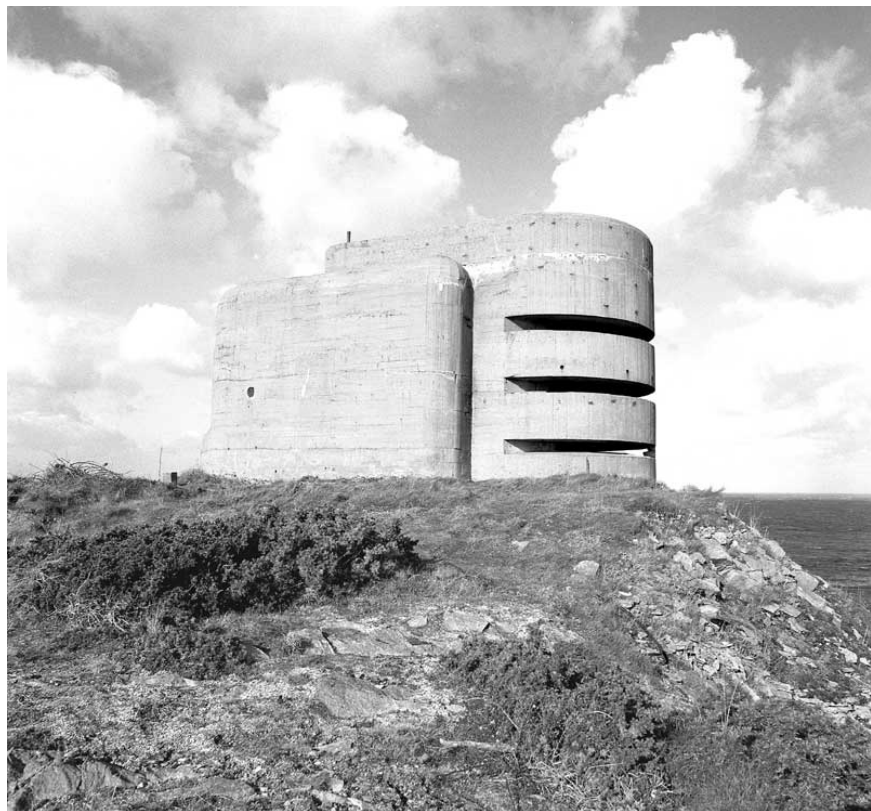
Fire Control Tower - Mannez Quarry Photo By Nick Catford
